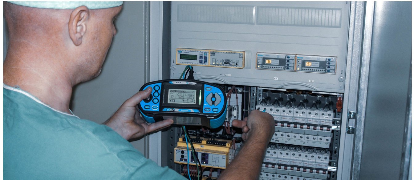
Testing protective RCDs in a mobile hospital. The whole such installation is isolated from ground.
