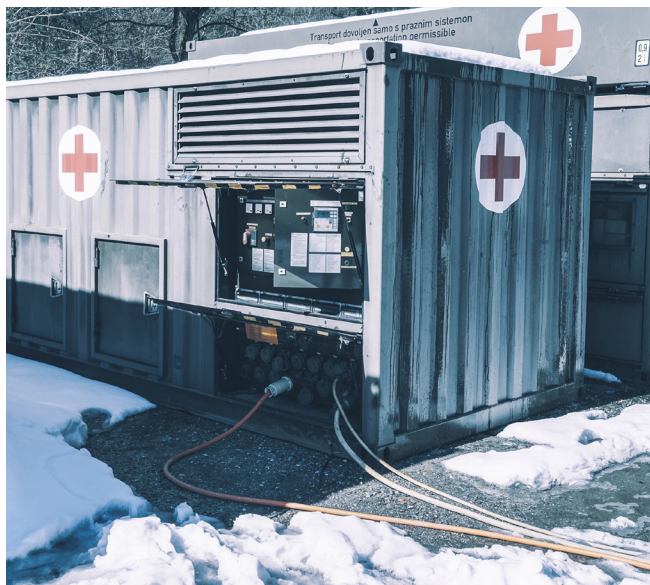
Electrical switchboard and inlets for army mobile hospital's power supply.
