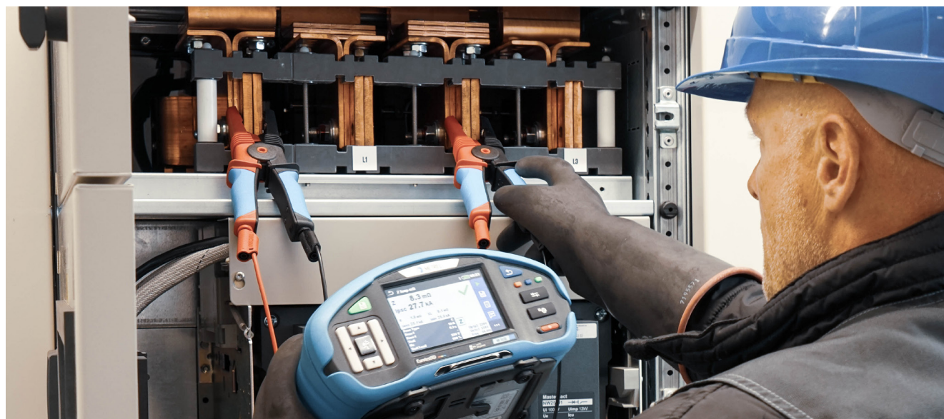
Measuring large busbars with Metrel kelvin clamps A 1593, MI 3155 and MI 3144.
