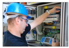
Unbalanced system means presence of IMD Insulation / ELM Earth Leakage / First Fault in Insulation and Single Fault Leakage Current.
